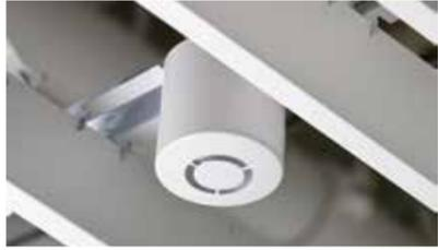
Throughout the bathroom facilities and back of house areas mySmart stand-alone motion sensors have been used. These sensors are not connected to the KNX lighting control solution as the needs for these areas are much simpler.
